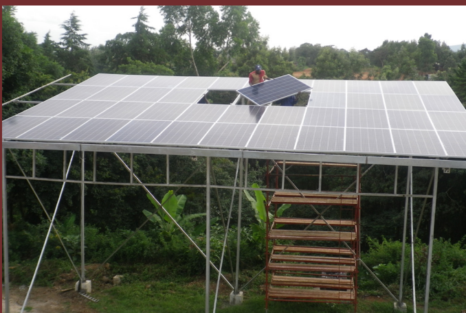
A technician completing the installation of solar photovoltaic plates
