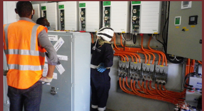
Engineers finalizing the installation of the solar power system
