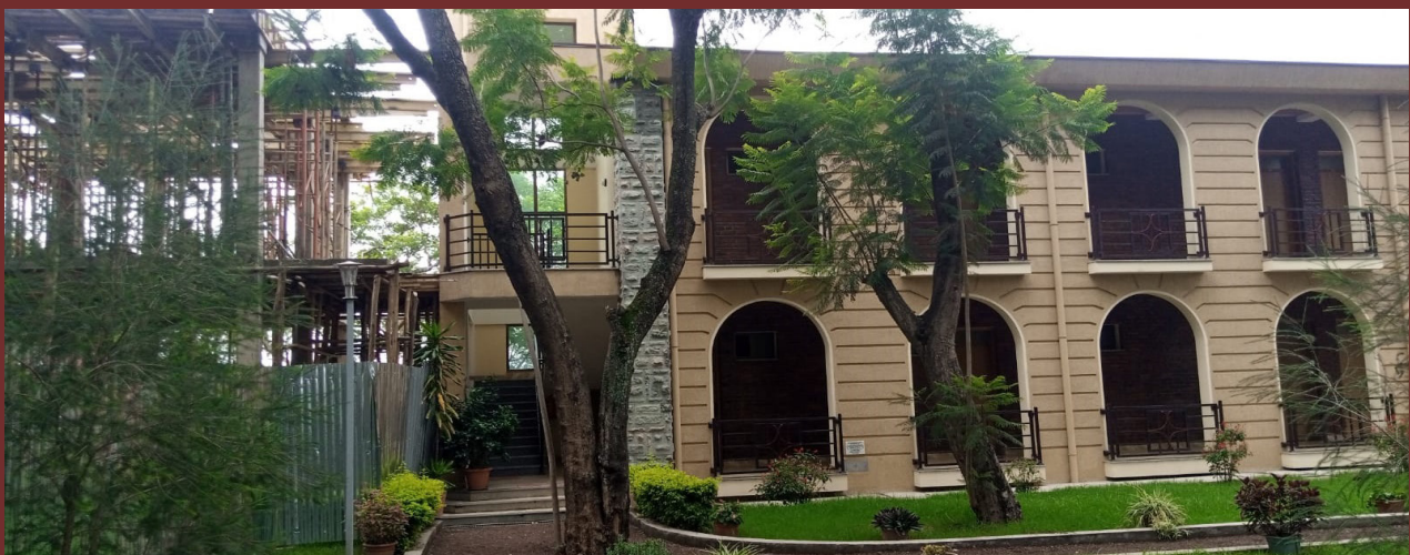
Galilee Jesuit Retreat Centre, Debre Zeit, Construction in progress.
