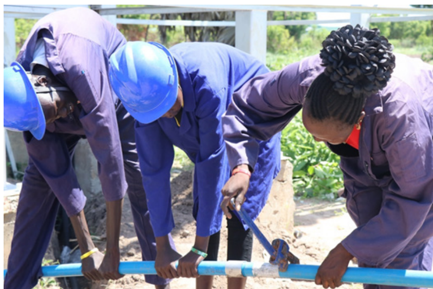
Plumbing practical at Loreto School, Rumbek, South Sudan.
