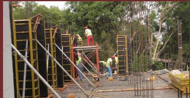
Preparing form work for the Columns of First Floor.
