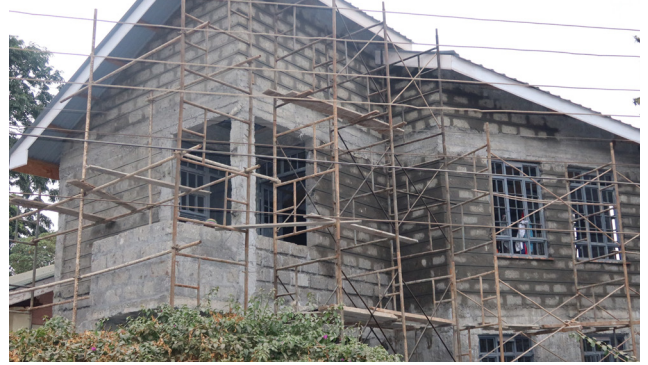
Construction of the new ultra-modern hall and library facility
