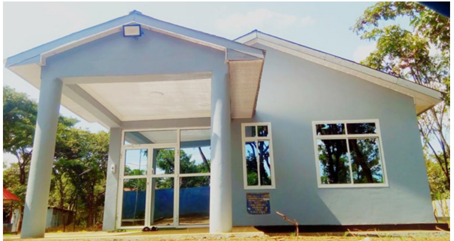
Newly Renovated Studio of Radio Kwizera in Kasulu in Kigoma. Photo by Marco – RK Reporter Kigoma town
