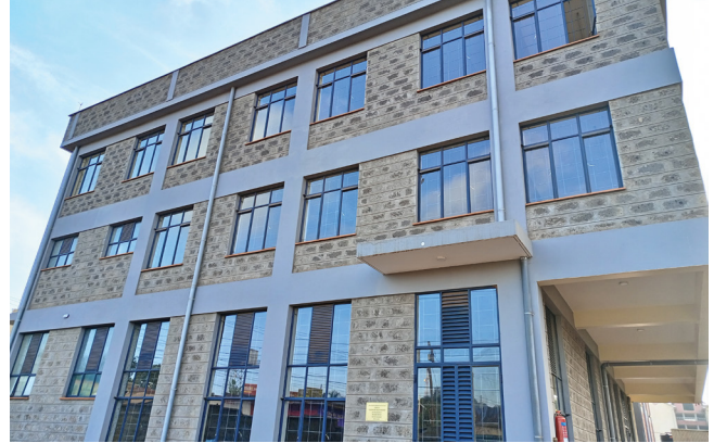
The new St Joseph Technical and Secondary complex Building which was funded by the Hungarian Government
